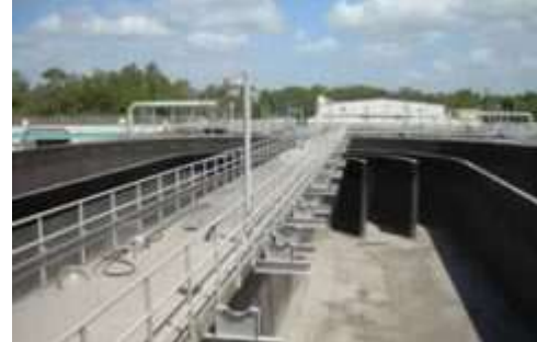
Eastern Water Reclamation Facility
